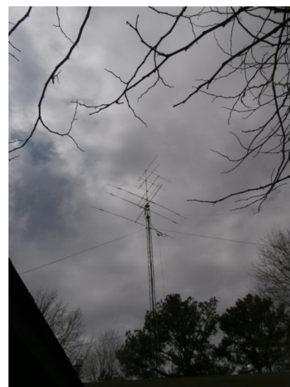
W5FWR antenna tower.
